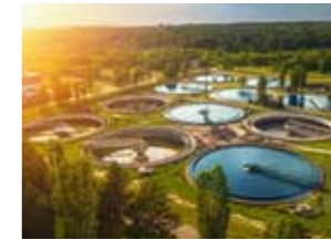
Sewage treatment plants
